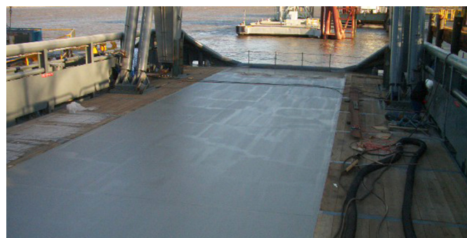
From top: Anchor impact areas, pipe deck protection, dropped object protection, and anchor handling pads
