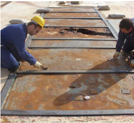
Figure 3. Oil storage tank P-770B: SPS no hot work repair.
